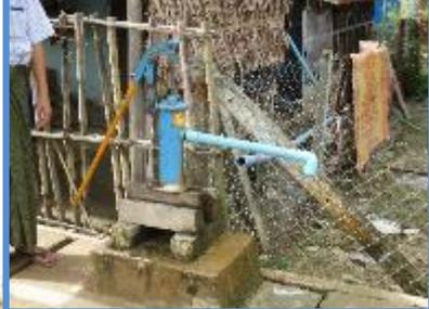
Hand pump isn't functioned. It is need to repair the washer.
